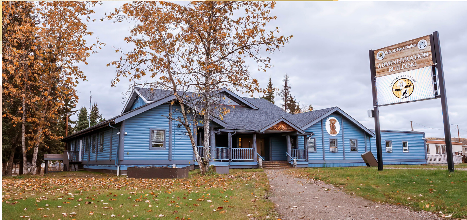
SFN Administration Building
